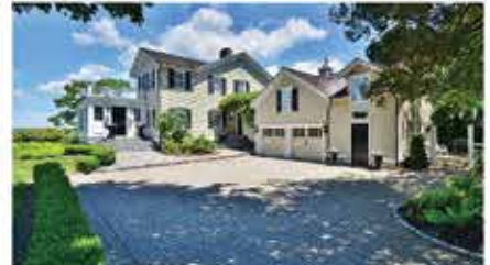
184 North Cove, Old Saybrook | Fabulous colonial was fully and meticulously restored and refurbished. Offered at $1,595,000
