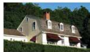
ESSEX PRISTINE 1790 CENTER CHIMNEY GAMBREL!
