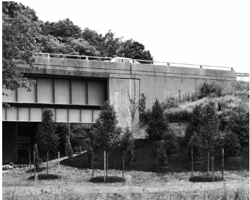
The Essex Foundation continued its gateway beautification work with juniper, Norway spruce, Canadian hemlock, and Chanticleer pear trees installed along the western slope of the Route 9 overpass between Routes 154 and 153.
